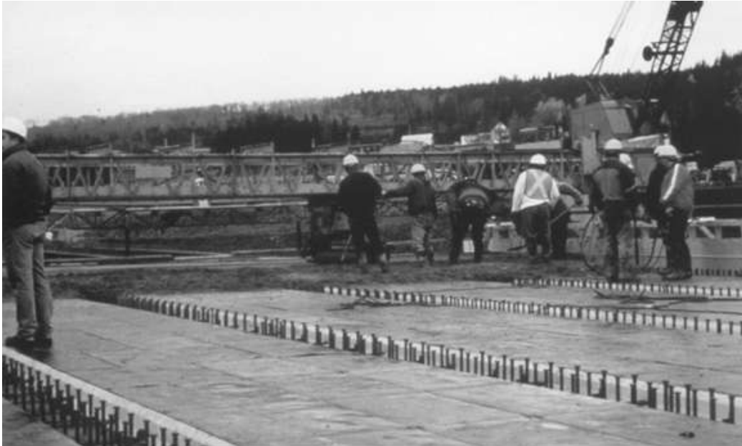
Figure 2.3 Pictorial view of the casting of the steel-free deck.
